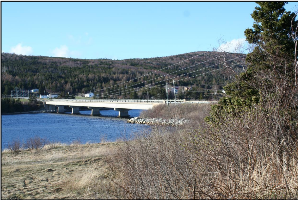
FIGURE 10: NEW GRAND BAY BRIDGE CONSTRUCTED IN 1983 (Photo taken May 10, 2023)
