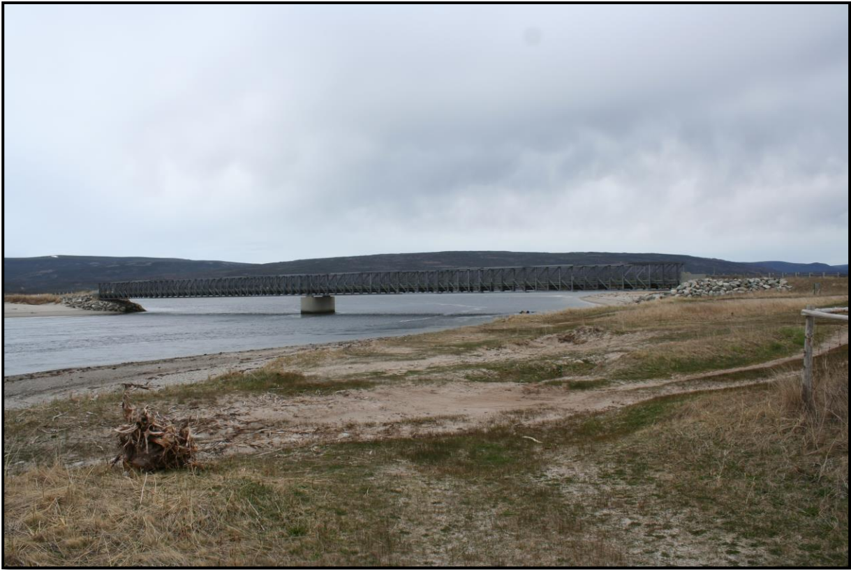
FIGURE 9: TEMPORARY “BAILEY” BRIDGE AT THE GUT COMPLETED IN APRIL 1978 (Photo May 9, 2023)
